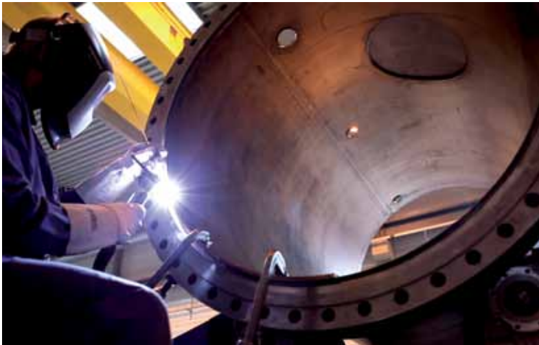
Welding a column using tantalum
