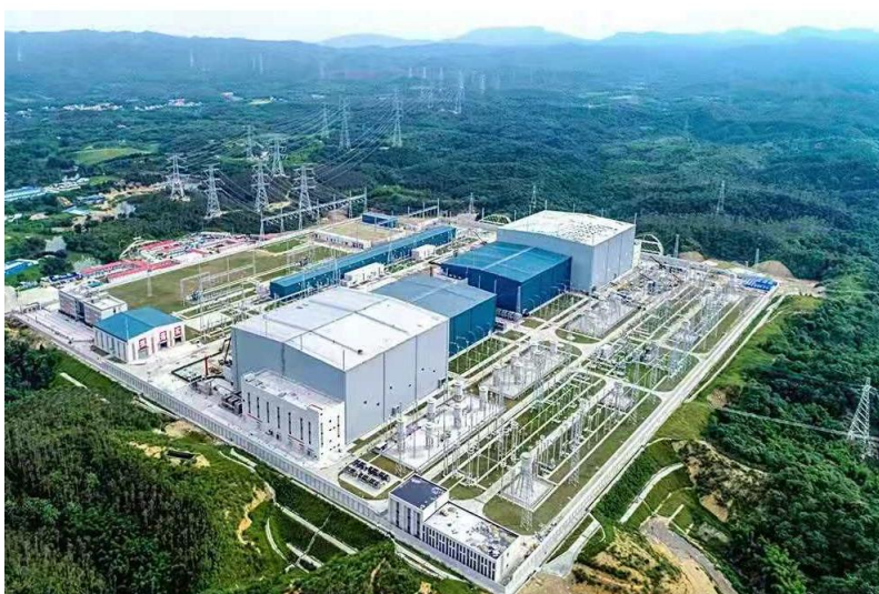
Power converter station in China
