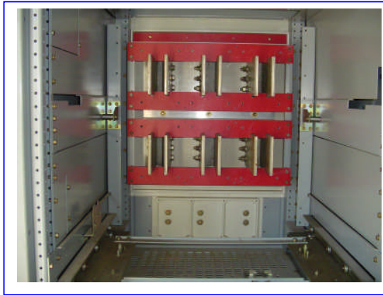
Fig. 6: The horizontal test setup was designed to simulate rear-fed equipment like this unit.
